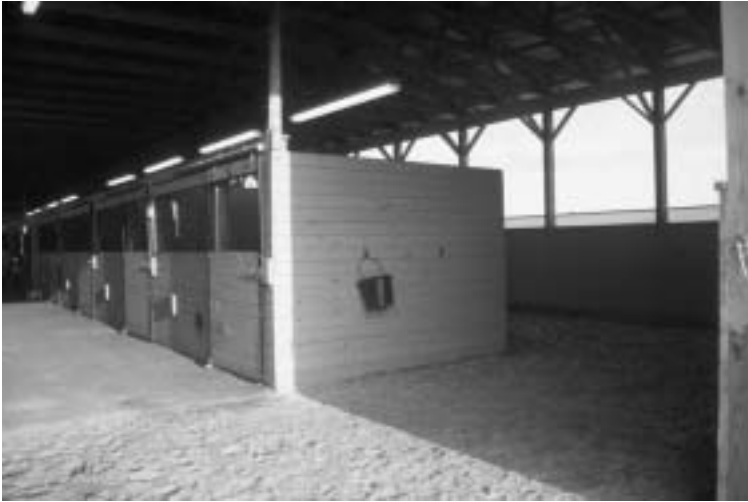
Figure 2.6. Island design puts stalls in the center of the structure with an exercise walkway around the entire perimeter. Shown is a portion of a racehorse stable with a center aisle stable surrounded by an exercise hallway with enough height so that horses can be ridden.
