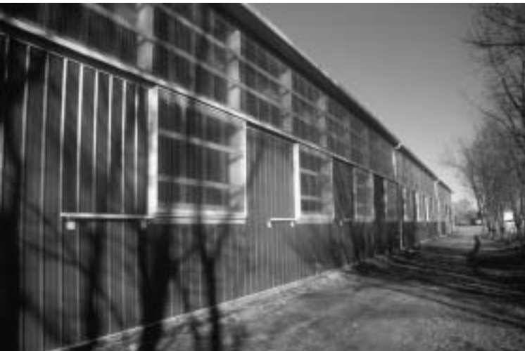
Figure 2.10. Maintaining a good interior environment of stables and arenas is very important. The interior environment should have adequate light level, which may be provided with translucent panels shown here. Admitting fresh air to arenas and stables is essential for horses and human handlers. Having panels like those shown here, which open for warm weather air exchange, is beneficial.
