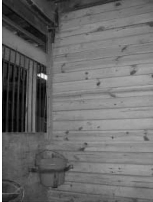
Figure 2.14. Labor-saving features and efficient routines are important because of the high labor demands of horse housing. This stall features a labor-saving overhead water line that supplies the bucket with water after a valve is manually activated.
