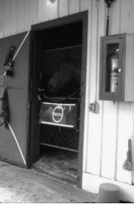
Figure 2.9. Horse facilities are built so as to ensure safety and minimize fire risk. Horse-proof hardware and construction is essential. Provide fire suppression tools as a backup to efforts to prevent fire ignition.
