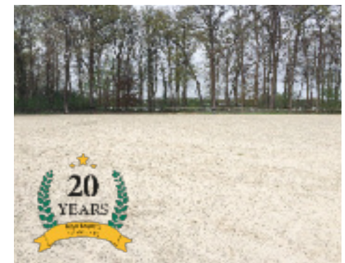
Footing layer over the OTTO-PerforatedMats
