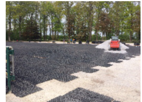
OTTO-PerforatedMats laid over a drainage layer
