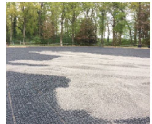
A fill layer goes over the OTTO-PerforatedMats
