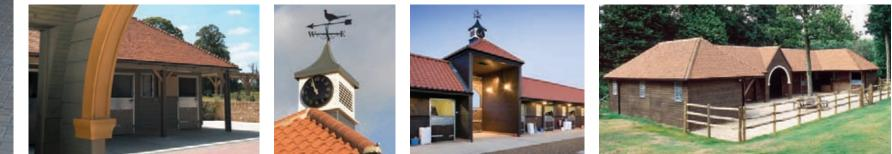
U-shaped dressage yard with 1.5m overhang and oak posts, 35° pitched roof finished in client's own tiles and clad in a deep feather edged boarding stained in "Slate Grey".
