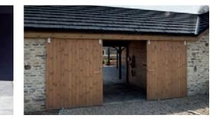
A professional pre-training yard with a 1.2m overhang, 30° pitched roof finished in pantiles and clad in tongue and groove shiplap boarding in "Spruce".
